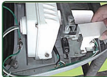
4 Loosen the screw and remove the hood of wiring box and top cover of wiring press.
