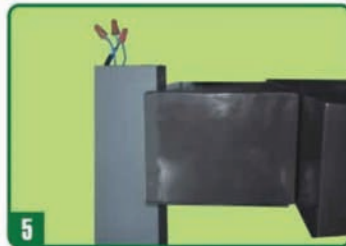
5 Connect all wire leads as per wiring diagram and tape the connection with water resistant glue.
