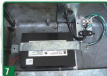
7 Connect the wire to the terminal as per the diagram.
